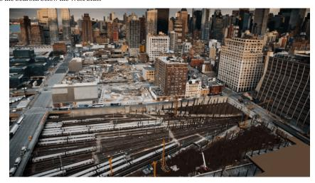
Once the caissons are in place, work will begin on a massively heavy, incredibly strong platform—a foundation perched on columns. This work will go piece-by-piece too, all to ensure the safety of the train drivers and the construction crews both:
