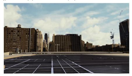
By the time the platform is complete, workers will have installed 25,000 tons of steel (more than half of the Williamsburg Bridge) and 14,000 cubic yards of concrete. It will weigh more than 35,000 tons. For comparison's sake, the bridge portion of the Brooklyn Bridge weighs around 14,680 tons.
