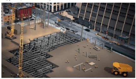
But the most difficult bit will come at the narrow neck of the rail yard. Here, the trains form a dense thicket of activity, and there's no room for massive caissons. Instead, crews will built a series of trusses across the rail yard:
