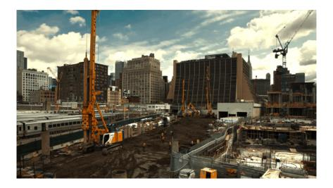
Builders have been doing this in NYC for ages—just look at the Brooklyn Bridge. A century later, this feat will be just as complicated: Because trains will continue to run through the yard, crews will sink the caissons in sections, avoiding the moving trains, drilling as deep at 80 feet into the bedrock below the West Side.
