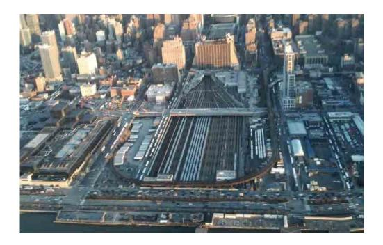
When the rail yard opened in the 1980s, its engineers were already imagining the day when a hungry developer would pave over it. So they left a small gap that runs around the edges of the yard—just enough space for structural members to be laid down without interrupting traffic. Think of it as an insurance plan for future city-builders.
